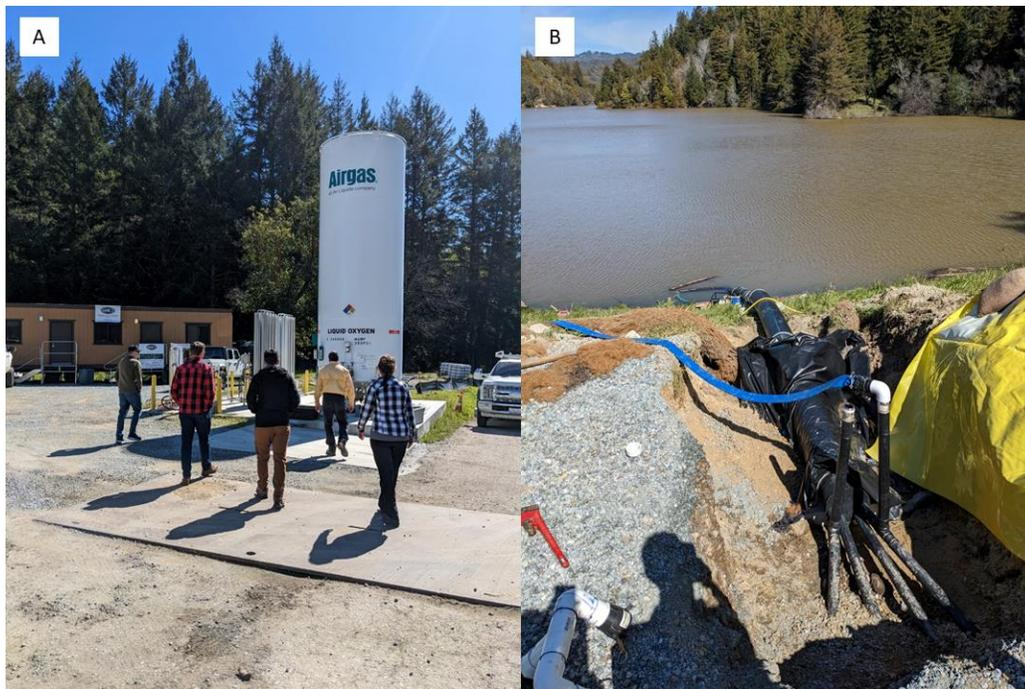
Figure 8.4.1.2. A) Onshore elements of a HOS installed in Loch Lomond, Santa Cruz, CA; B) Pipes connecting the onshore elements with the diffusers in the lake
